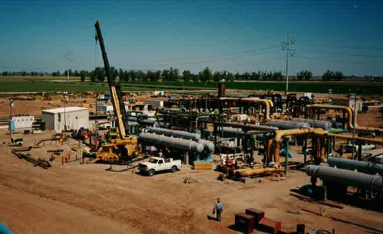
Heber SIGC under construction, back in the Polaroid days.
